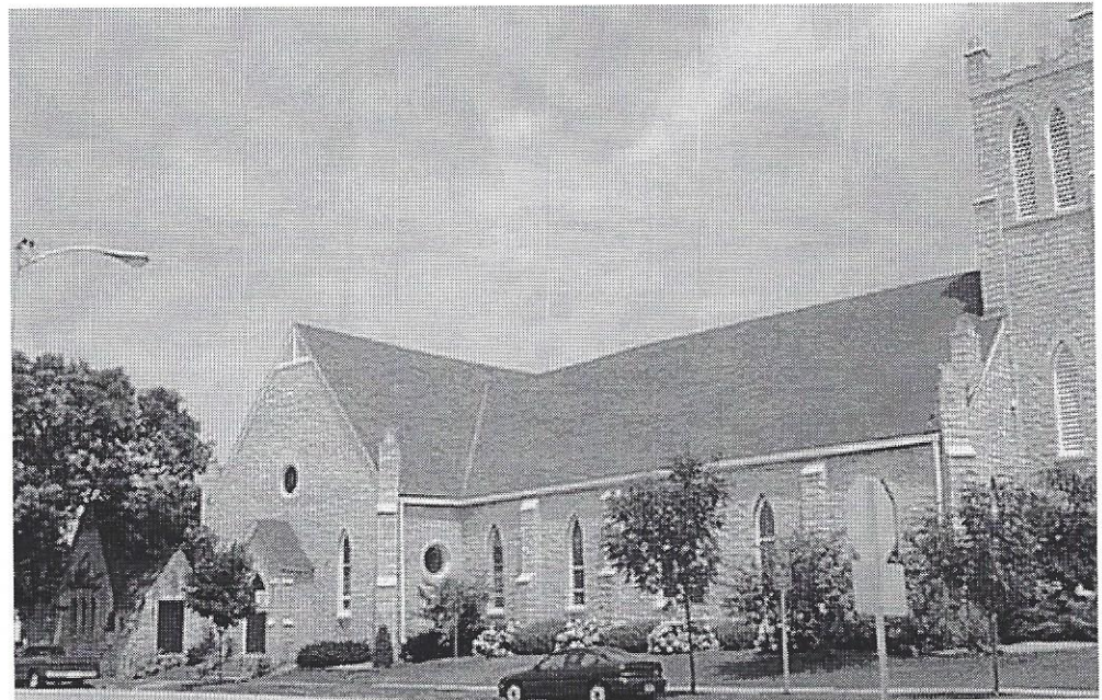
west side - pointed arch stained glass windows, pilastered stone detail, round windows in cross gable corner towers
