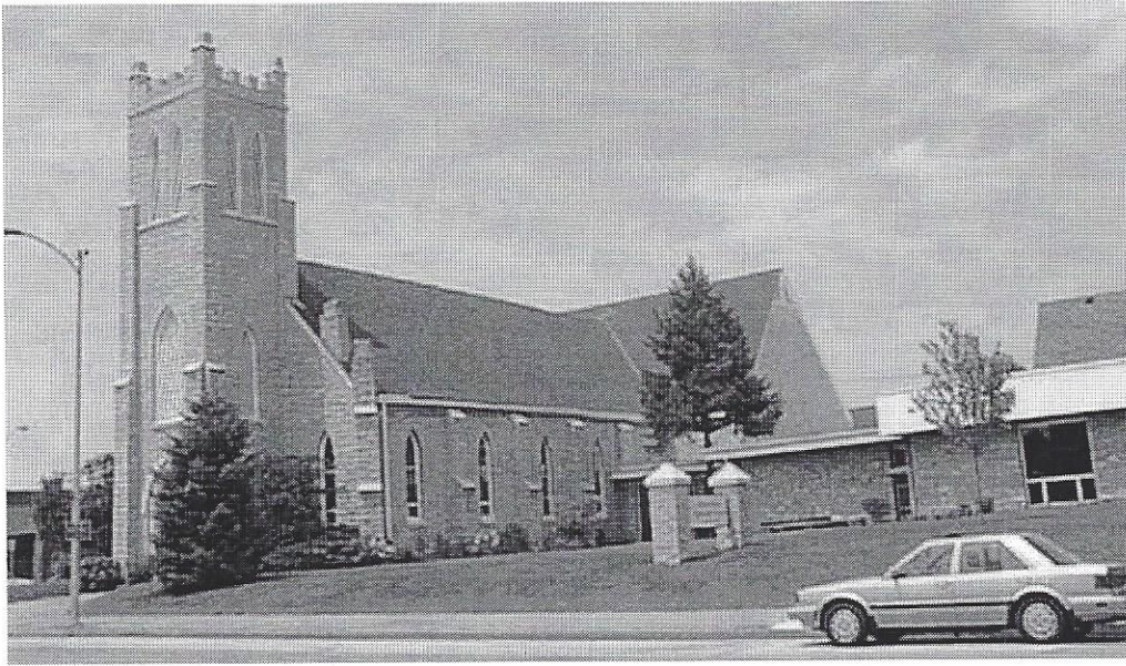
east side - pilastered stone details, pointed arch stained glass windows, stone cross gable, (1866 addition), corner towers
