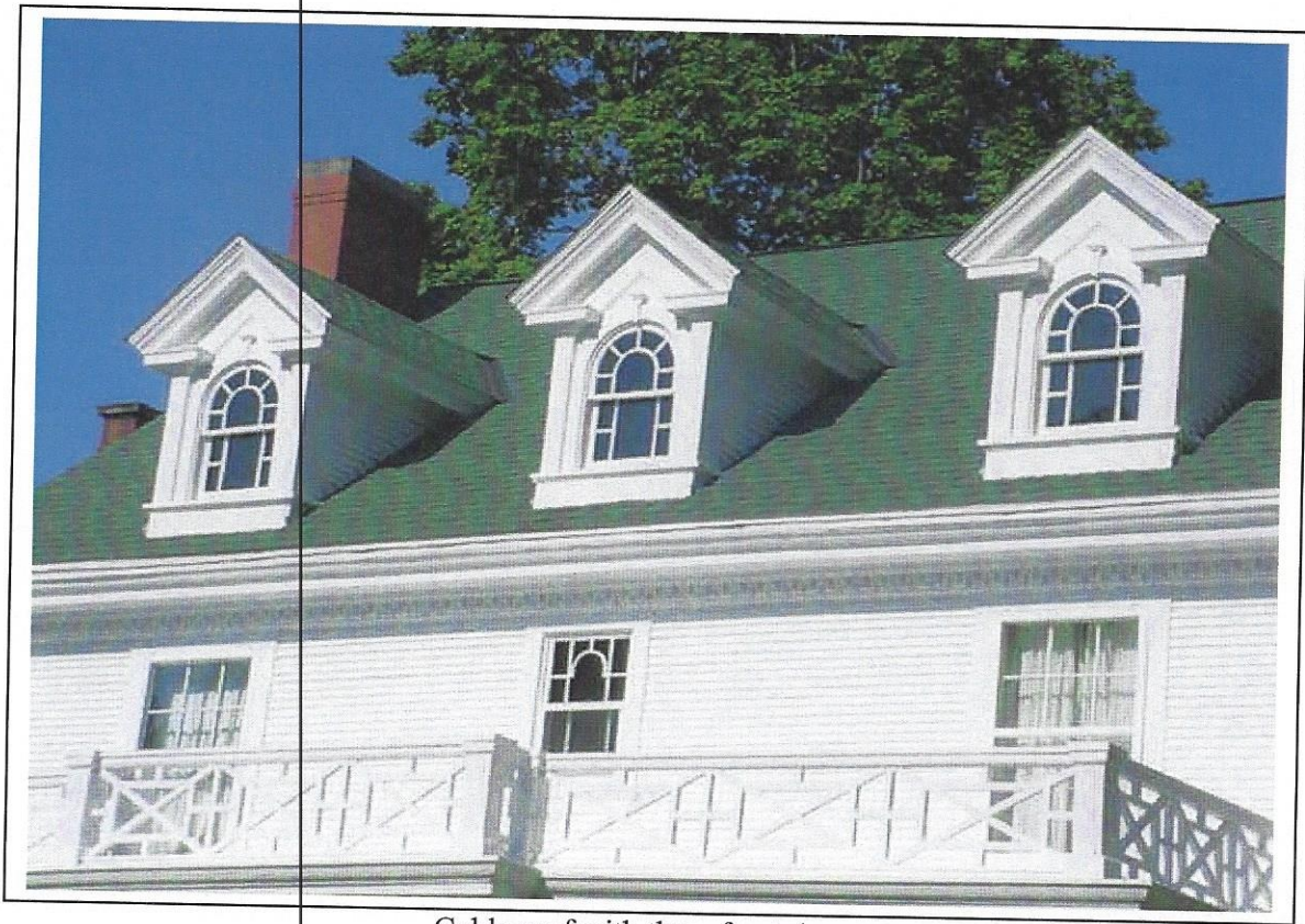
Gable roof with three front dormers
