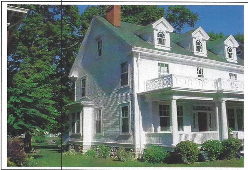
Southeast corner showing chimney, stone foundation, and projecting window on the first-story
