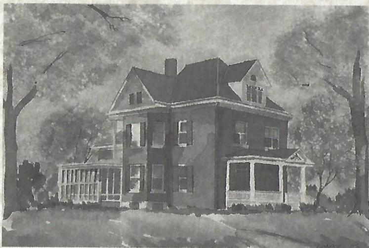
1420 Kentucky The John F. C. and Selma Schott House Free Classic Queen Anne Style • 1901 Architect: Frederick C. Ledebrock Current Owner: Carolyn Kolodziej
