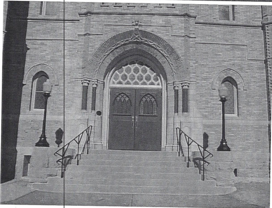
Main east entry - double doors, brick arch indentation detail, stone detailing, stone base, columns, foundation light supports
