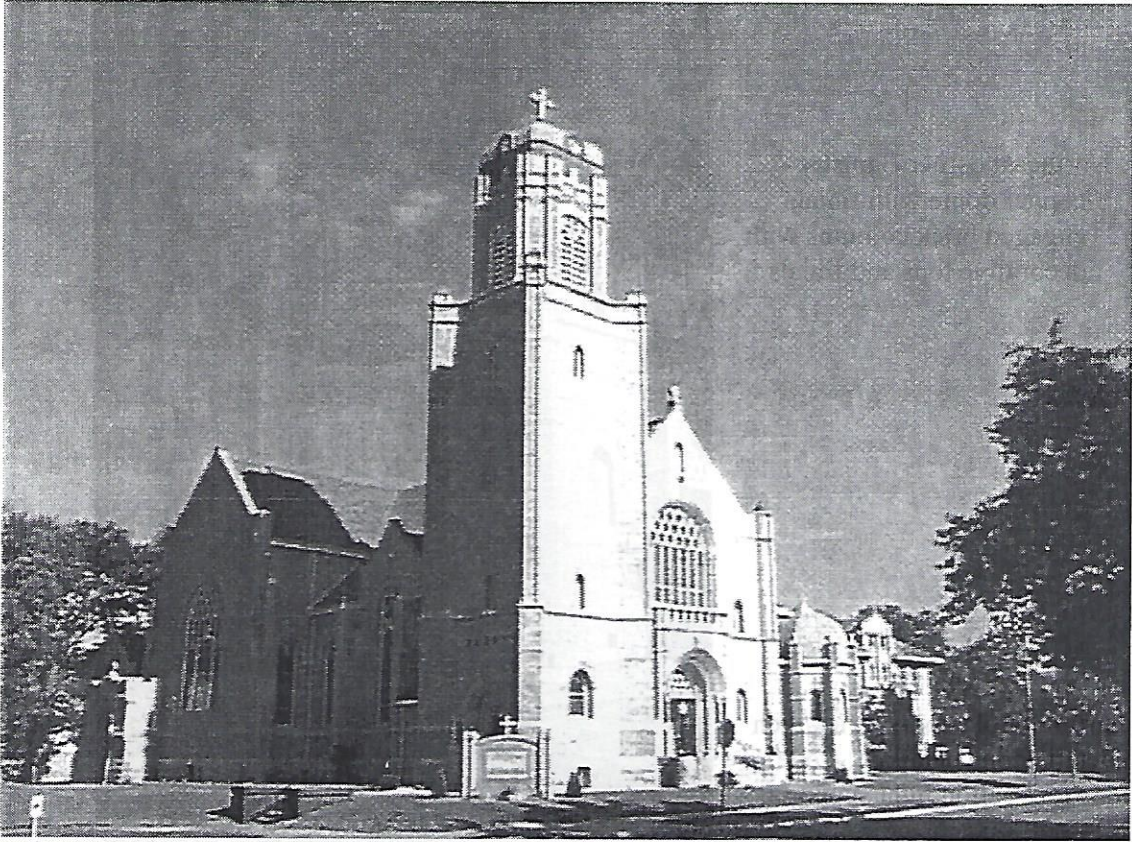
Southeast corner bell tower - small arch windows on sides, decorative top, south entry, gold cross
