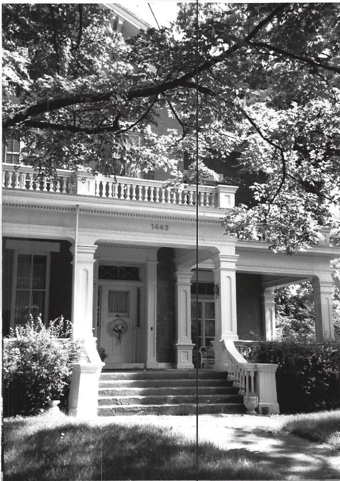
Detail of two-story front porch entrance with Classical elements, square carved columns, balustrades at both levels. Colonial Revival front door has top and side lites.
