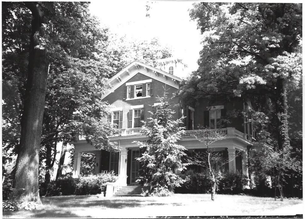
View from street, facing north. Cupola is visible.
