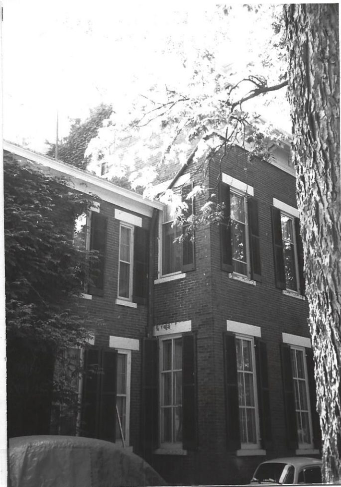
Northwest corner of main volume, the rear of the house most likely was a later addition, accounting for the change in window levels.
