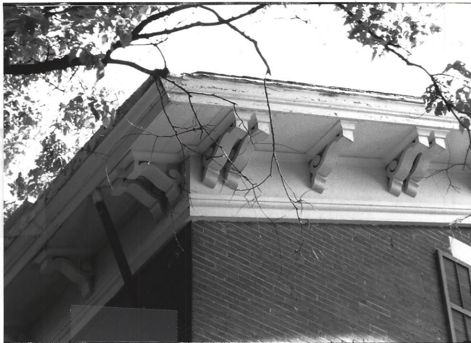
Detail of carved scroll brackets supporting cornice.
