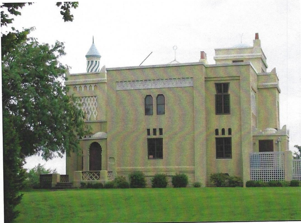
General view, 2008 -- east façade.
