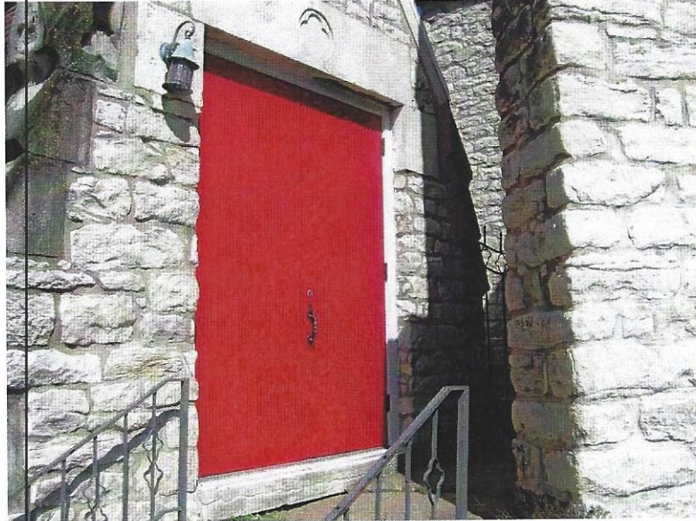
Side entrance w/double doors on west, St. John's Parish Church 701 Hampshire
